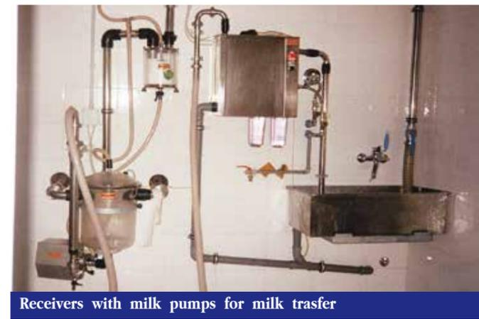
Receivers with milk pumps for milk trasfer
